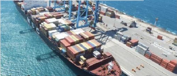
Fortaleza International Deep Water Port
